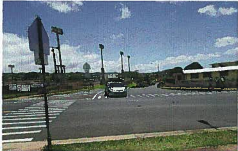
The pedestrian crossing across Ulune is 100 feet wide. A pedestrian would be exposed to traffic for over 22 seconds, while holding back motorists, where as a more compact design brings the exposure time down to 10 seconds.
