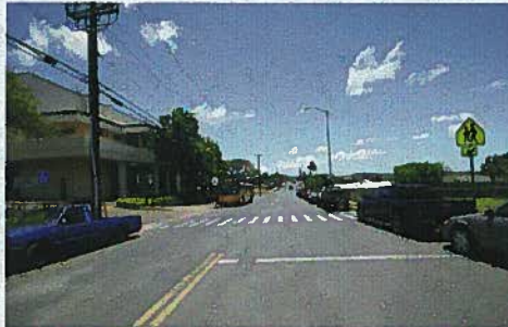
Parking needs to be enforced through design so that vehicles cannot park in between the advance stop bar and marked crossing to improve sight lines for both motorists and pedestrians.
