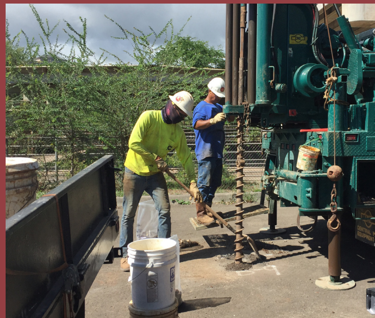
Soil borings at Animal Quarantine Station (Geolabs, August 2020).
